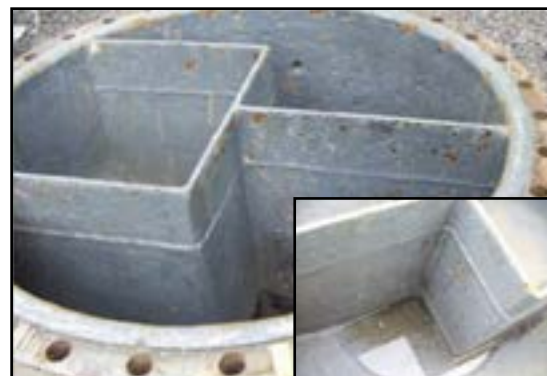
After coating with ARC 855 and ARC S2
